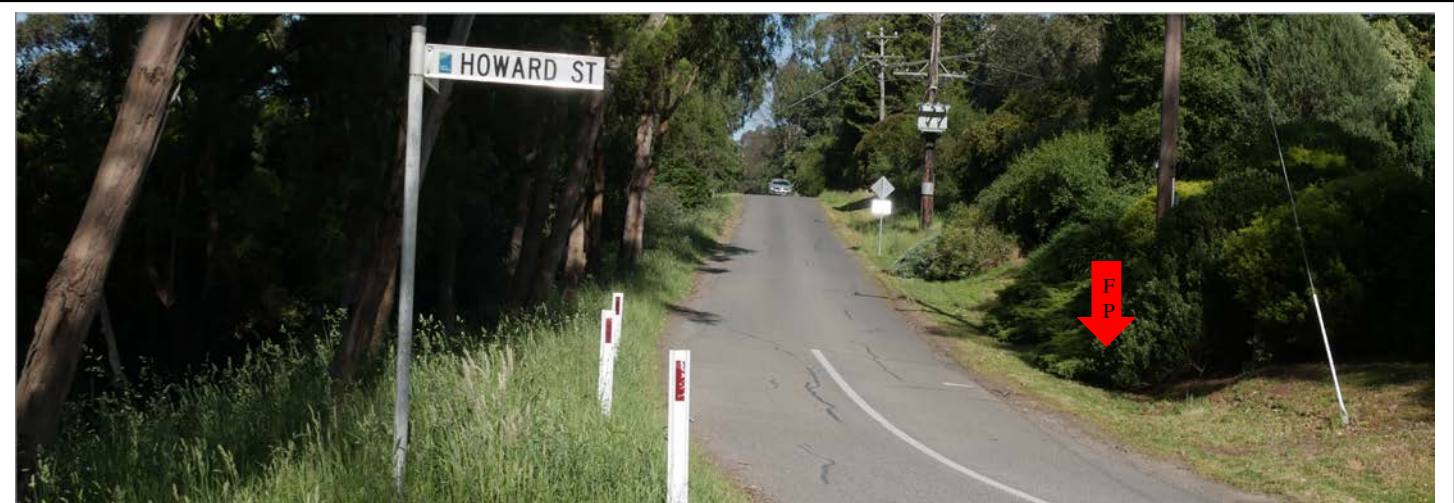
Photo 8 Seymour Rd across the road of Lot 1 is a fire Plug
